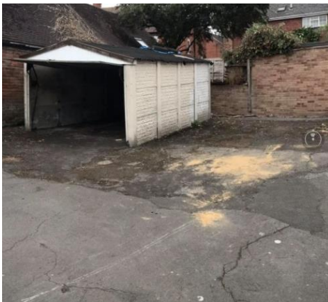
Here's the garage, emptied and ready for demolition!
